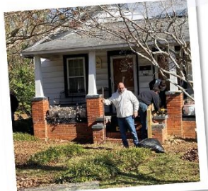
Raking the yard and building handrails for elderly people JENSEN USA
